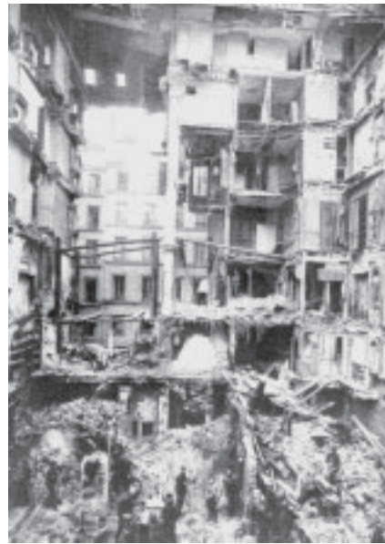
Damaged inflicted on Paris building by one “Big Bertha” shell fired from 75 miles away.
