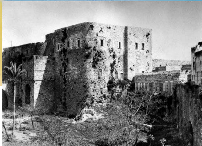
Exterior of the prison cell where Bahá'u'lláh was first confined in 'Akká.
