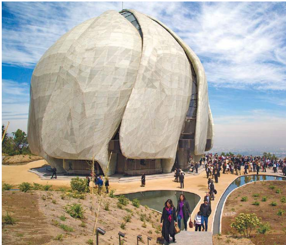
Bahá'u'lláh's instruction to make Bahá'í Temples "as perfect as possible in the world of being" has inspired advances in architecture, design, and engineering. The Bahá'í House of Worship for South America, completed near Santiago, Chile, in October 2016, required the development of a new approach to casting glass to create nine wing-like sheaths with the strength of stone and the luminescent quality of glass.
