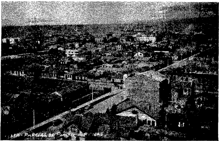
View of the city and harbor of Punta Arenas, where the first Bahá'í Local Spiritual Assembly in this southern tip of Chile was established on April 21, 1941.
