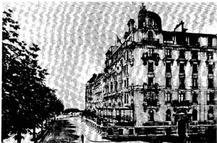
International Center, 37 Quai Wilson, Geneva, Switzerland, site of Bahá'í International Bureau and offices of Bahá'í European Teaching Committee
