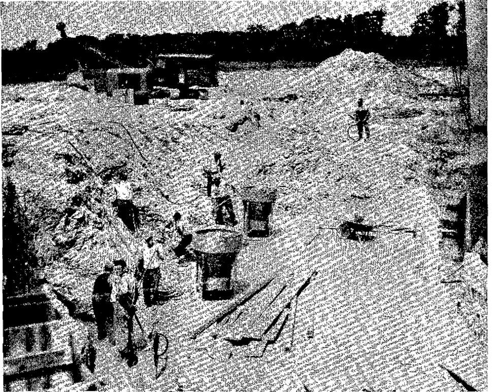
Excavating the foundations.
