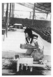
A Bahá'í using a very simple machine to make adobe bricks for the Guaymi Cultural Centre, built by Bahá'í sin 1985; Boca del Monte, Panama
