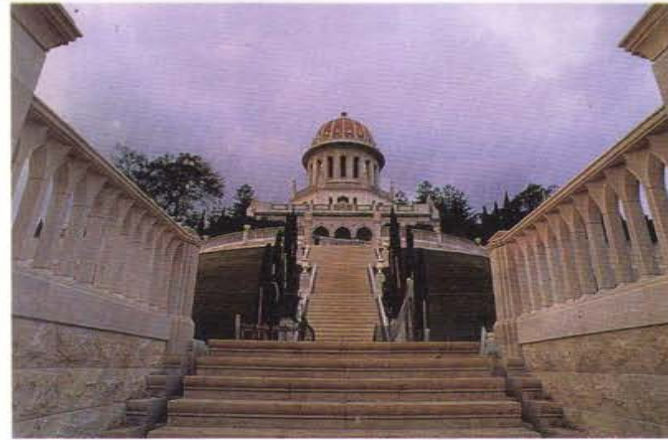
A view of the finished terraces below the Shrine of the Báb.
