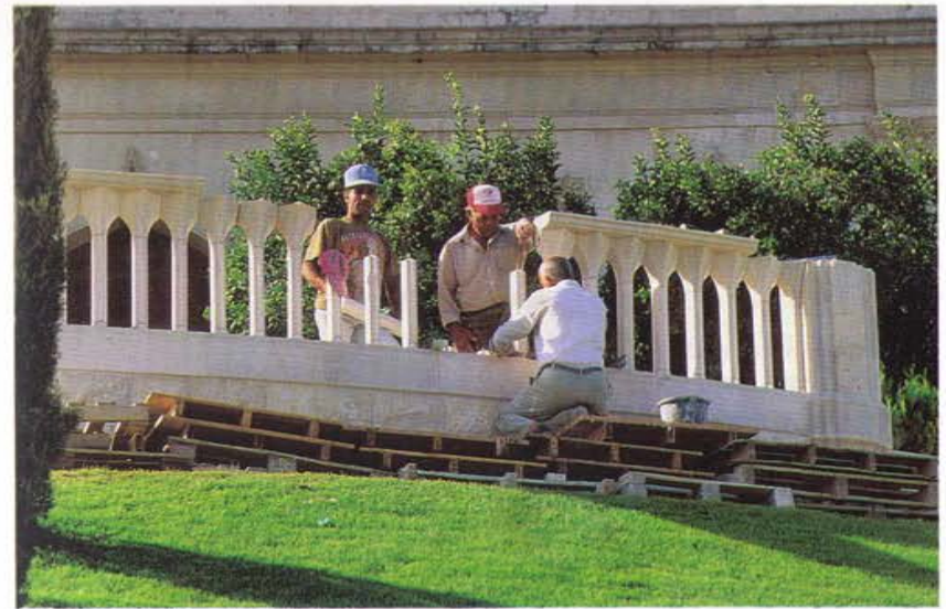
Balustrades from Israeli stone cut and polished in Italy comprise one of the principal adornments for the terraces of the Shrine of the Báb.
