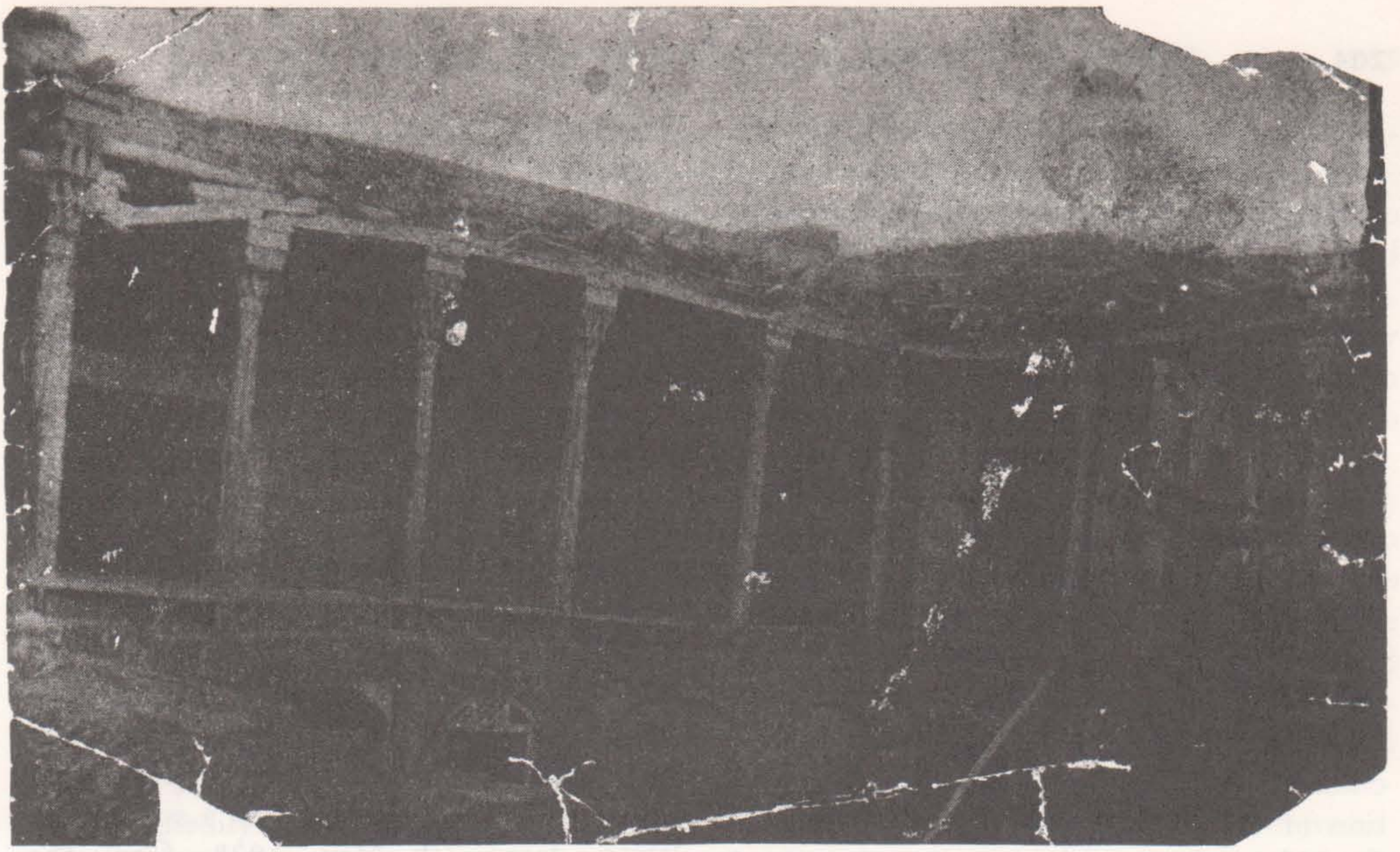
A view of the inner courtyard of the House of Bahá'u'lláh in Baghdád.
