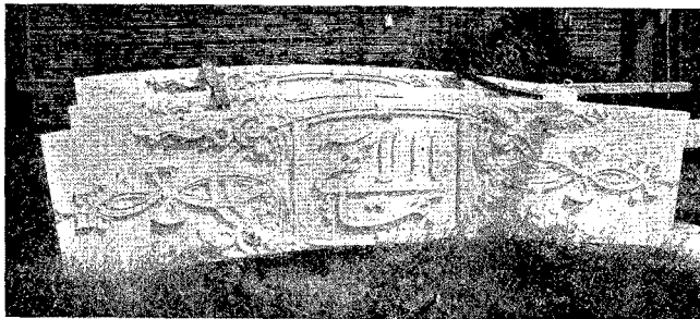
Castings of the Greatest Name which go over the nine Main Entrances of the Temple. The Persian inscription means "O Thou Glory of Glories." The first of these sections were placed in position in November, 1940.
