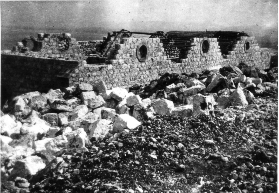
The Shrine of the Báb under construction in the time of 'Abdu'l-Bahá
