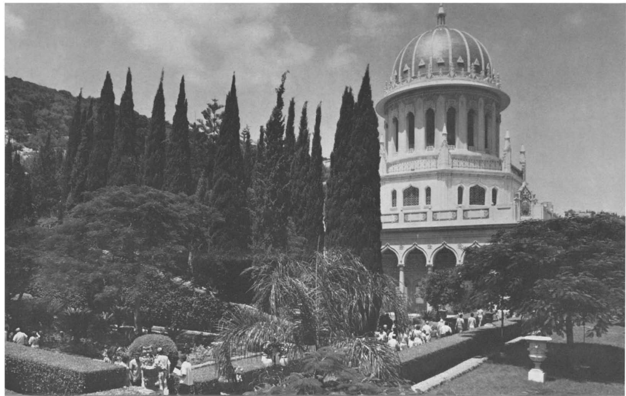
THE SHRINE OF THE BÁB ON MT. CARMEL The superstructure erected under the guidance of Shoghi Effendi
