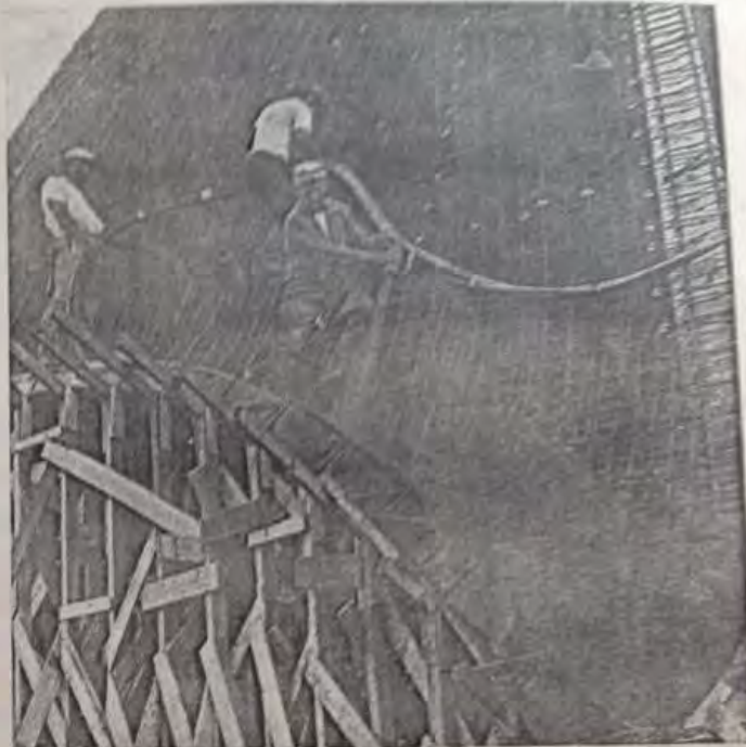
Early stages in the guniting process on the dome.
