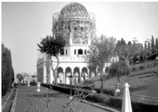
The dome and drum of the Shrine of the Báb take shape over the completed octagon and colonnade, 1952. Haifa, Israel. © Bahá'í International Community. Bahá'í Media Bank
