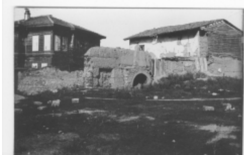
Photograph taken in Edirne during a visit in Oct. 1933 by noted Bahá'í teachers Martha Root and Marion Jack. Root described this scene as 'a portion of the old foundation wall and the great old fireplace where the cooking was done at the Amr'u'llah Big house in Adrianople.' The house, located across the street from the famous Sultan Salim mosque, was Bahá'u'lláh's residence at the time of the final break between Him and Mírzá Yahyá. On 10 Mar. 1866 Bahá'u'lláh withdrew to the House of Rida Big, which is still standing. National Bahá'í Archives, United States.
