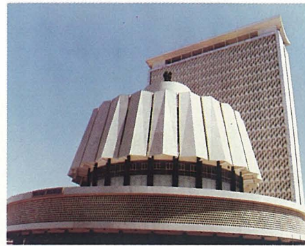
Above : New Council Hall for Maharashtra in Bombay.
