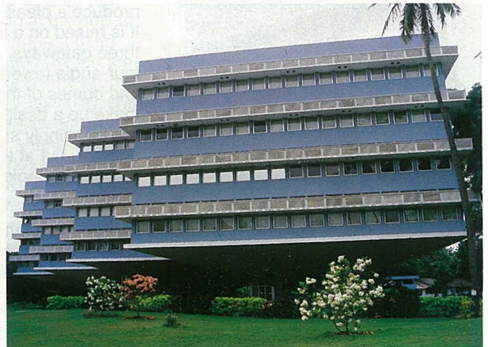
Headquarters of ECC Construction Group of Larsen & Toubro Limited in Madras.
