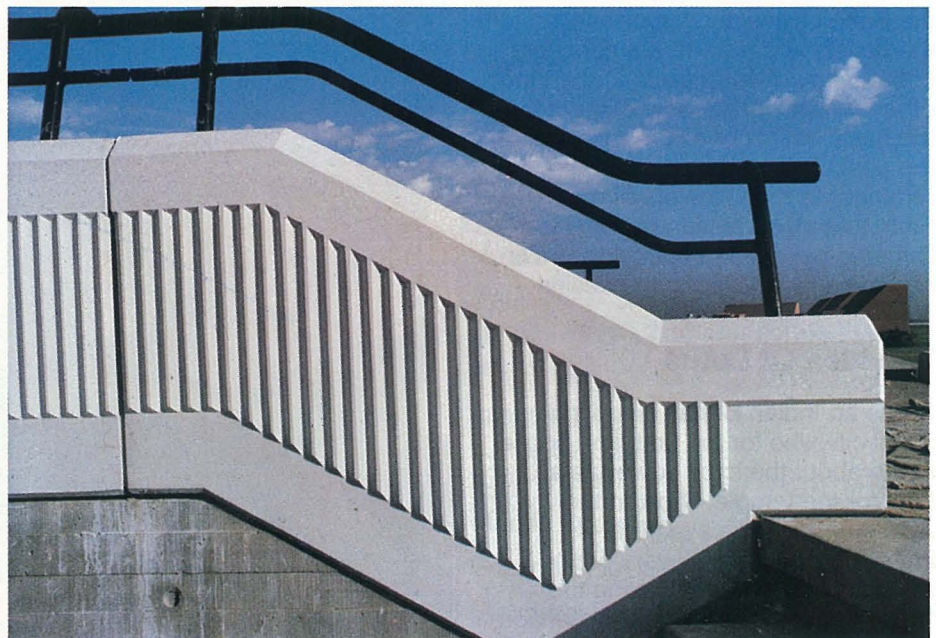
Precast concrete balustrade with handrail, showing architectural patterns.
