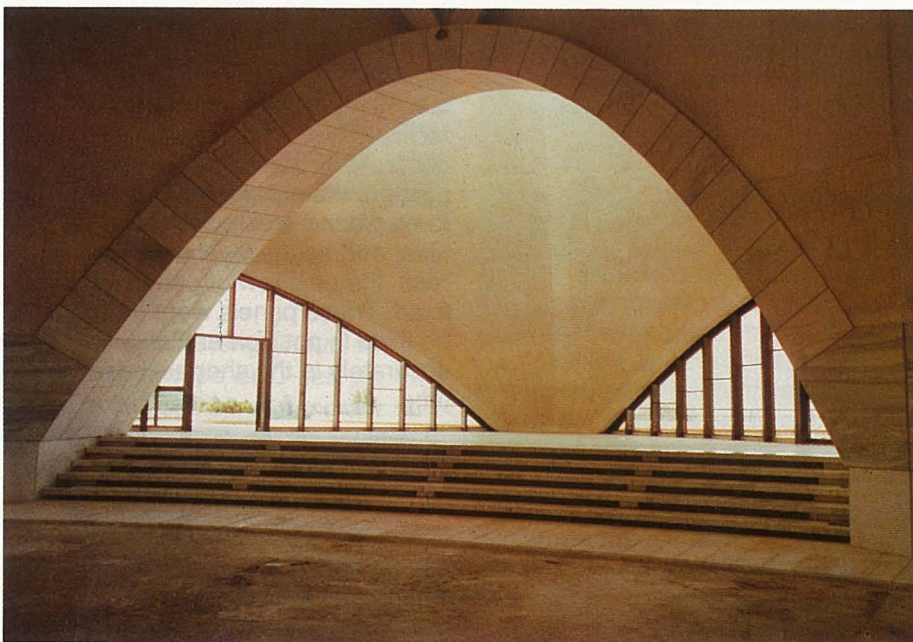
The Baha'i temple — showing part of the assembly hall.
