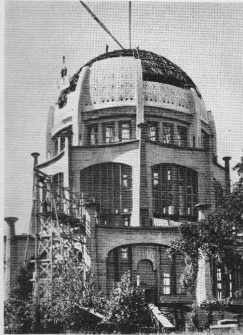
Units of exterior ornamentation applied to the superstructure form a permanent outer surface or shell.
