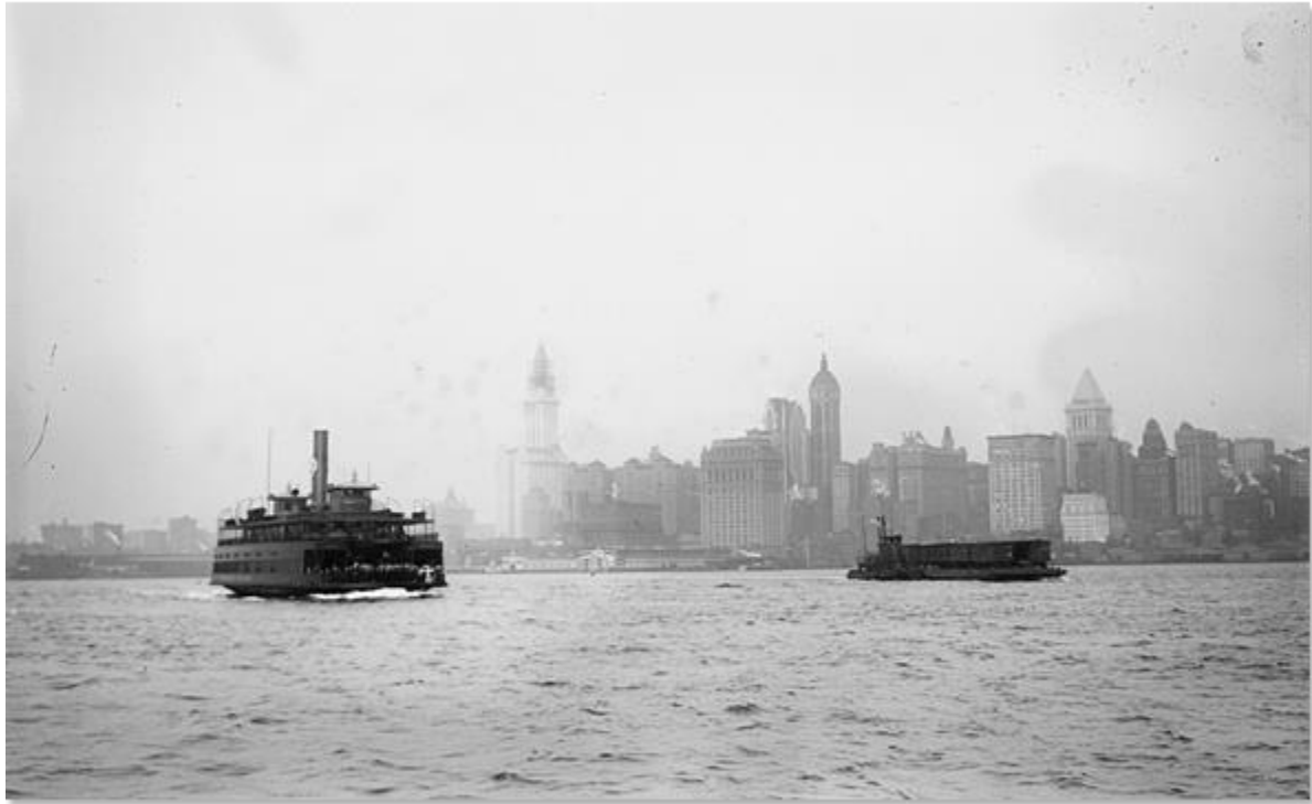
Lower Manhattan from the mouth of the Hudson River. The Woolworth Building is still under construction in late 1912. (Bain Collection, Library of Congress)
