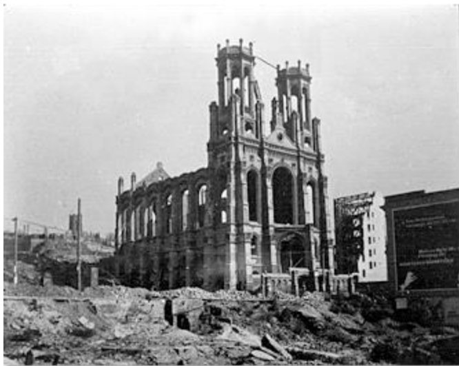
Temple Emanu-El gutted by fire after the 1906 earthquake. (U.S. Geological Survey)
