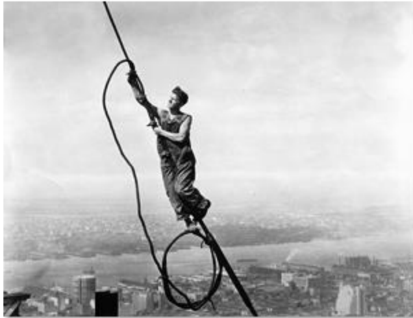
"Icarus Atop the Empire State Building," by Lewis Hine, circa 1930. A worker fastening steel cable to hold a derrick in place prior to lifting steel girders and other steel parts at the top of the skyscraper. (Underwood & Underwood)
