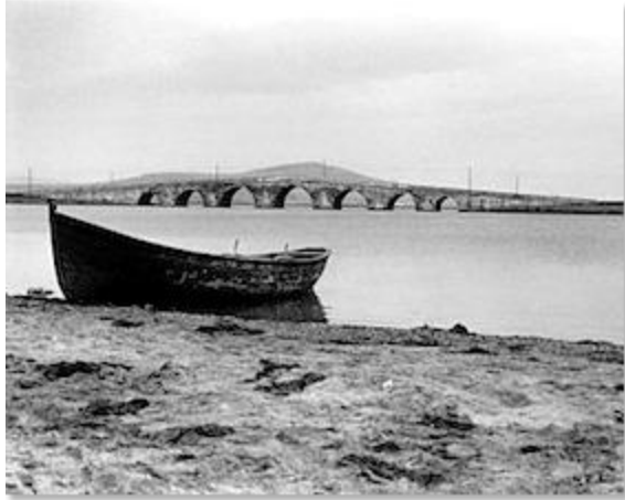
The bridge at Büyükçekmece, Turkey, which Bahá’u’lláh crossed on his way from Constantinople to Adrianople in December, 1863. (Bahá’í International Community)
