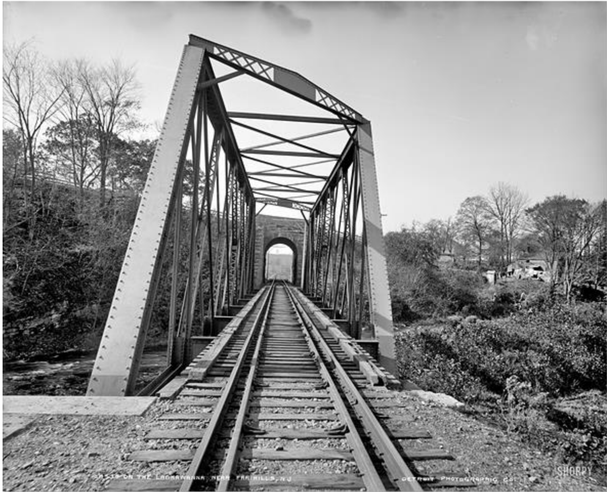
A railway bridge over the Lackawanna River, New Jersey, circa 1900. (Detroit Publishing Company)
