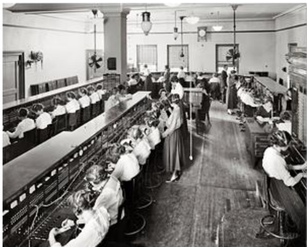
Switchboards of the Chesapeake & Potomac Telephone Co. in Washington, DC, about 1919. (Harris & Ewing)
