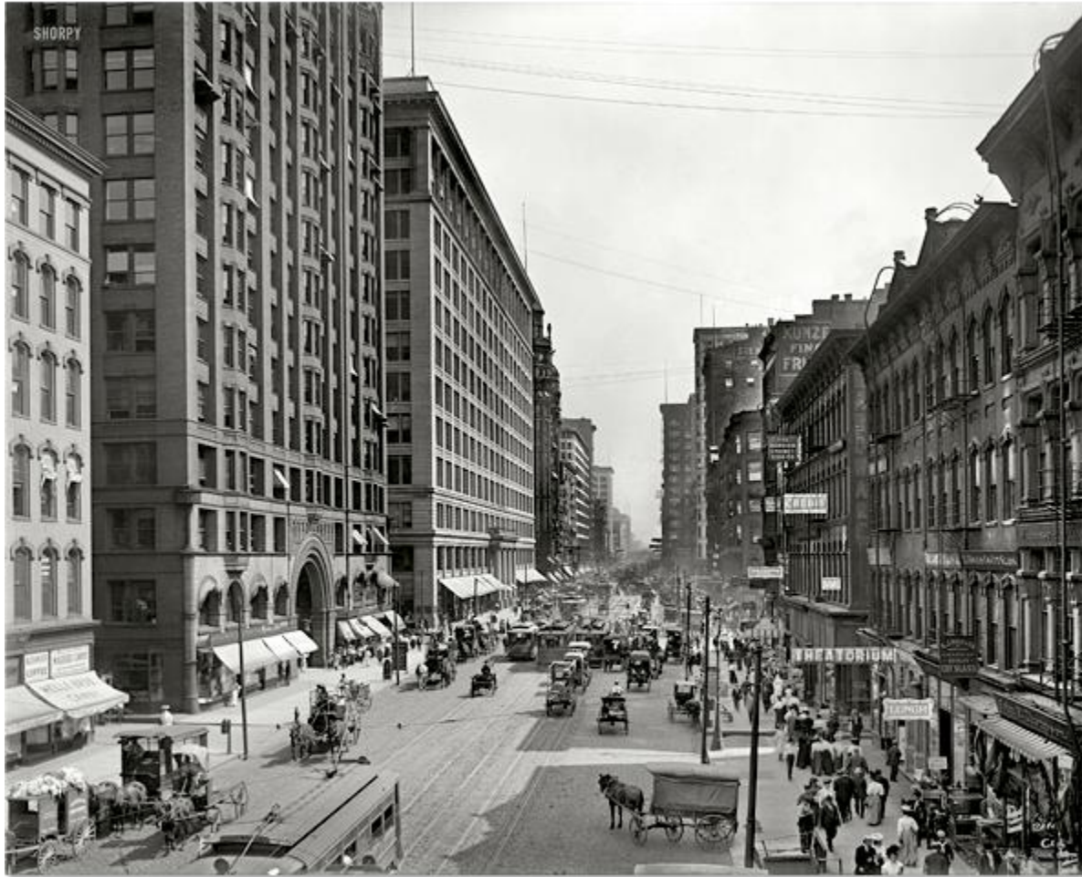
Looking south down State Street from Lake in downtown Chicago, 1907. The second building on the left is the Masonic Temple, where 'Abdu'l-Bahá spoke to the Bahá'í Temple Unity convention on May 1, 1912. (Hans Behm/Shorpy)
