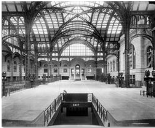
The main concourse at Pennsylvania Station, New York, c. 1910. (Detroit Publishing Co.)
