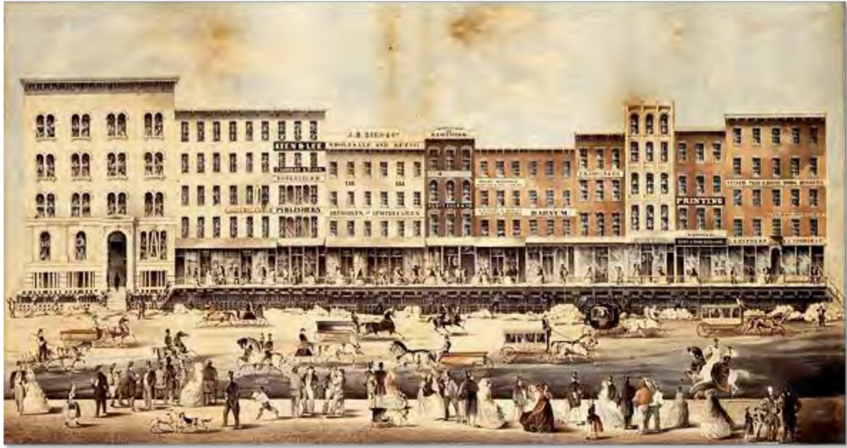
In 1860, an entire block of Lake Street in Chicago was raised five feet off the ground while shopkeepers and patrons continued to go about their business. (Wikimedia)
