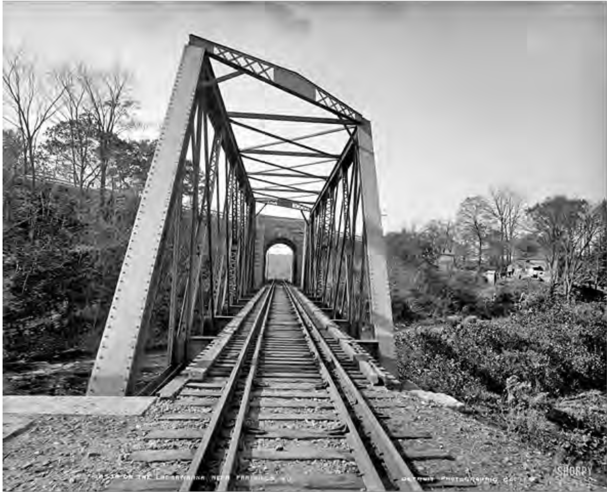
A railway bridge over the Lackawanna River, New Jersey, circa 1900. (Detroit Publishing Company)
