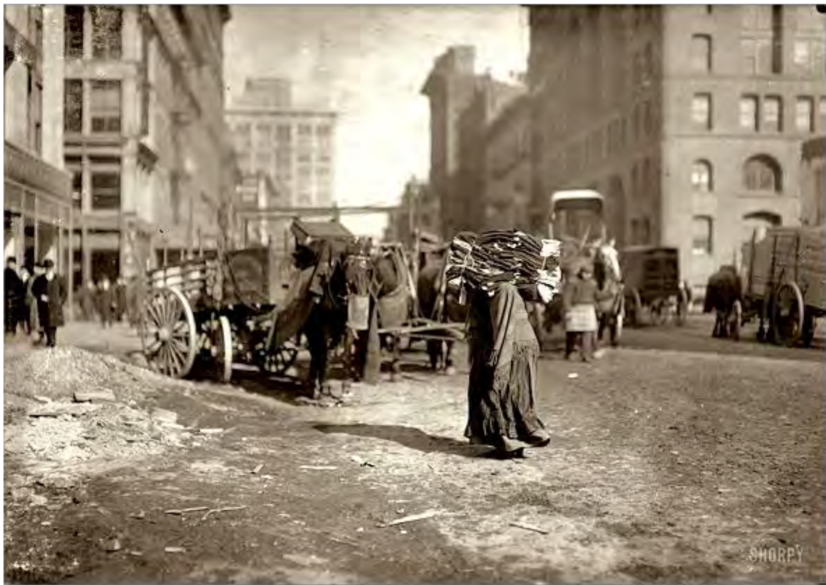
"The breaking point. A heavy load for an old woman. Lafayette Street below Astor Place." This photograph, taken by Lewis Hine in February 1912 for the National Child Labor Commission, depicts an old lady near Broadway in Lower Manhattan stooped by the weight of the pile of fabric she carries. (Library of Congress)
