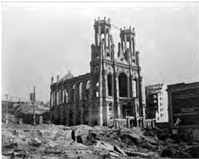
Temple Emanu-El gutted by fire after the 1906 earthquake. (U.S. Geological Survey)
