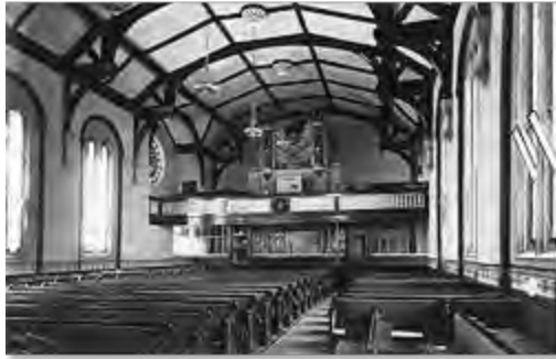
Inside the Church of the Messiah, Montreal, about 1870. (Alexander Henderson/McCord Museum)
