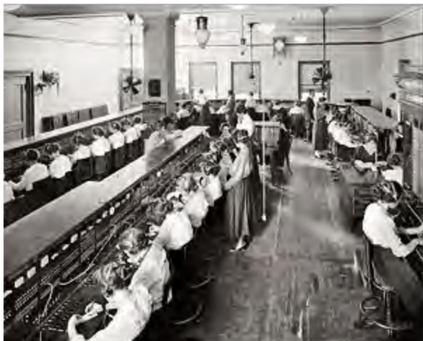
Switchboards of the Chesapeake & Potomac Telephone Co. in Washington, DC, about 1919. (Harris & Ewing)
