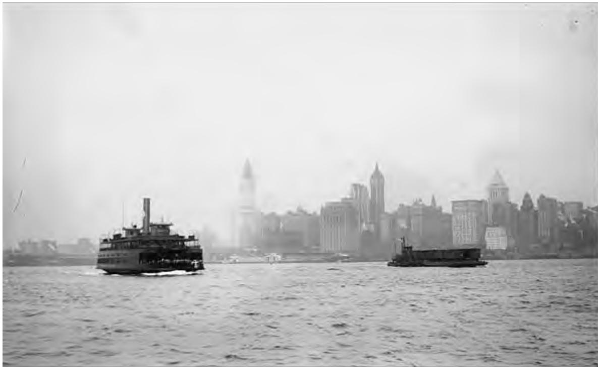
Lower Manhattan from the mouth of the Hudson River. The Woolworth Building is still under construction in late 1912. (Bain Collection, Library of Congress)
