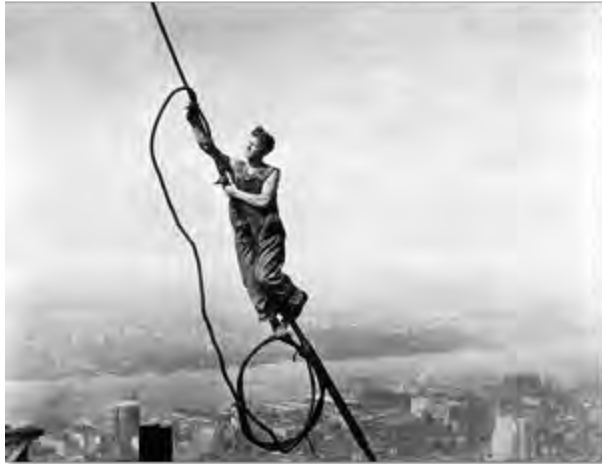
"Icarus Atop the Empire State Building," by Lewis Hine, circa 1930. A worker fastening steel cable to hold a derrick in place prior to lifting steel girders and other steel parts at the top of the skyscraper. (Underwood & Underwood)
